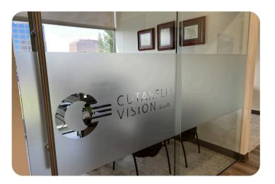
Specialized types of window & wall films designed to enhance various aspects of building performance and occupant comfort. Most films are made from a polyester base material, which is a durable and flexible polymer that can be easily manipulated into thin sheets.
